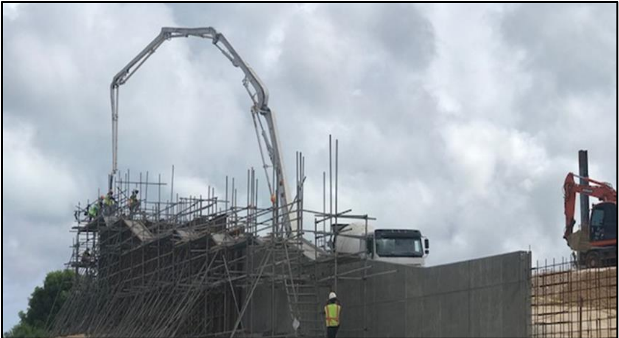
New U.S. Courthouse under construction.
