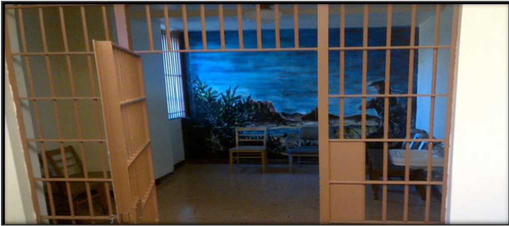
Outdated prisoner holding cell, built in the 1930's. Wooden chairs, porcelain plumbing fixtures, and glass light fixture are not maximum security and could be used as weapons.
