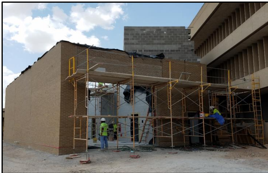
Vehicle sallyport construction.
