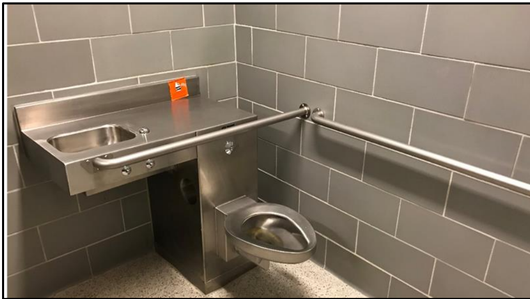
Finished product: accessible prisoner toilet.
