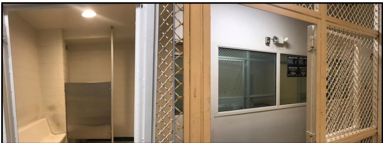
Cellblock prior to renovation.
