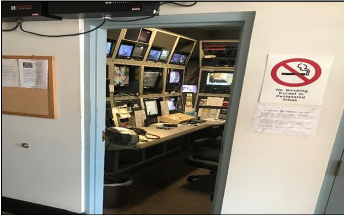
Command and control room along prisoner movement path (prior to renovation)
