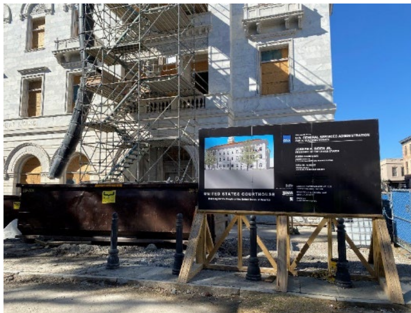
Savannah, GA – Historic courthouse restoration underway.
