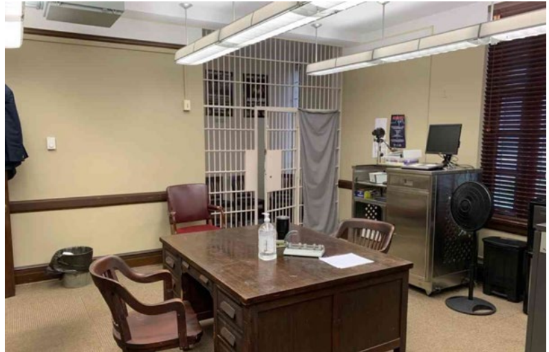
El Dorado, AR (planned renovation) – Antiquated USMS office dating to 1900s. Holding cell, prisoner processing, and DUSM space in one area. Each should be located separately.
