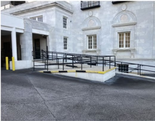
Augusta, GA – Prisoner delivery area to without enclosed vehicle sallyport. A current Capital Security Program project including a sallyport is underway.
