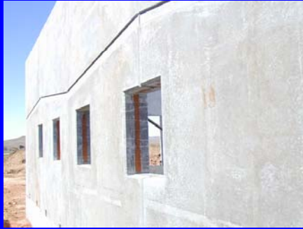
Facade In Construction
