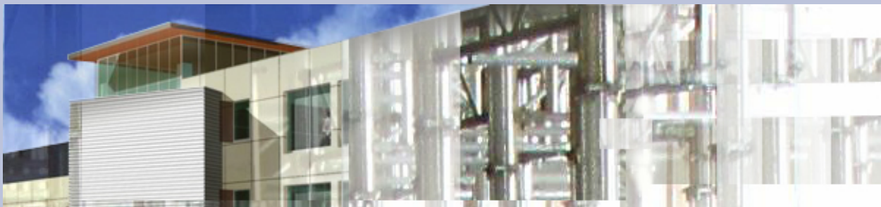
Radiological Laboratory/Utility/Office Building, Chemistry and Metallurgy Research Replacement Project Los Alamos National Laboratory Image
